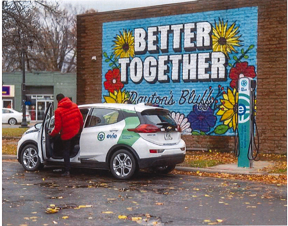
An example of ROW charging infrastructure (Credit: HourCar)
