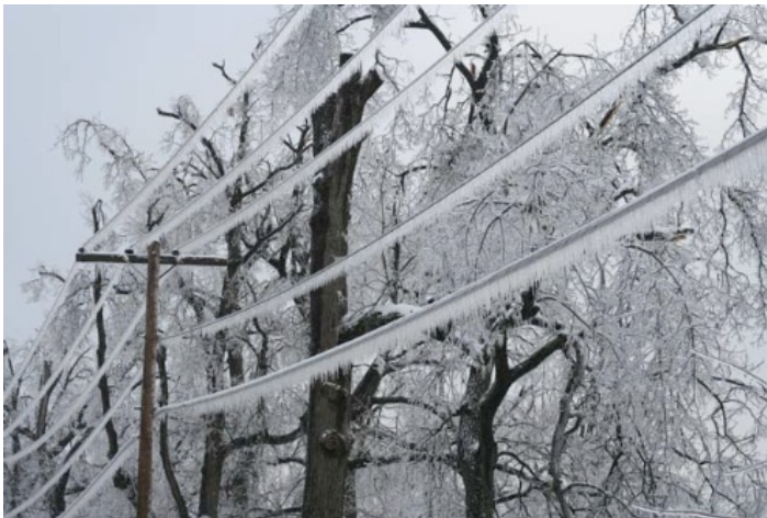
Figure 3-22 Ice Covered Power Lines
