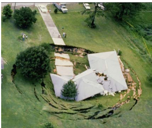
Figure 3-17 Home Swallowed by Land Subsidence
