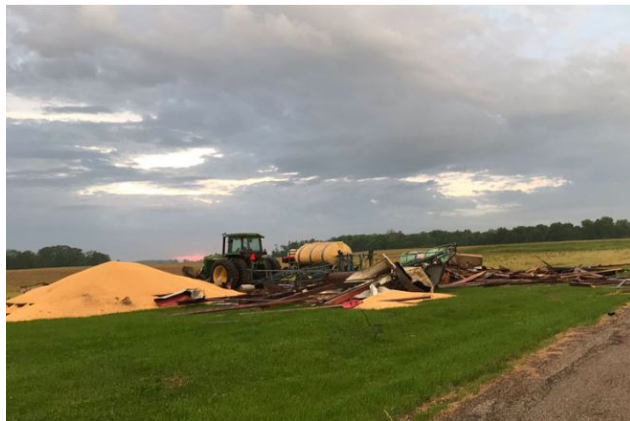
Figure 3-19 May 2019 Tornado Damage
