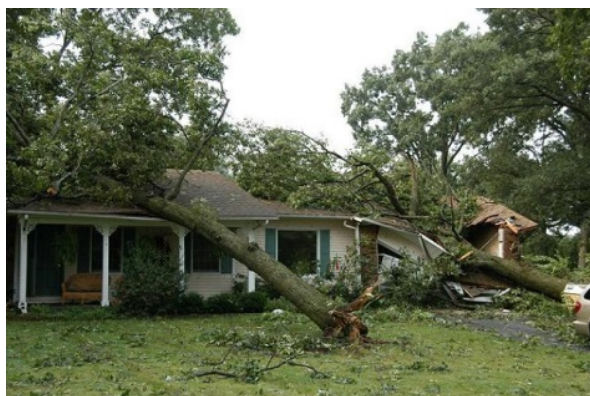
Figure 3-16 Home Damaged During Windstorm
