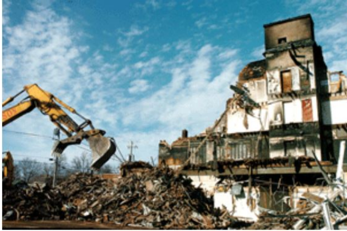
Figure 3-13 Demolition of Centennial Towers (Rochester Sentinel)
